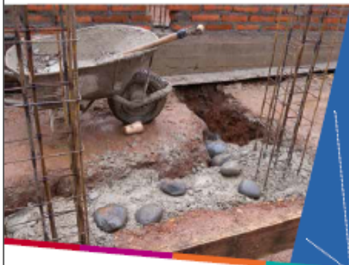
Image 1: Tie-column reinforcement cages extending from foundations of a new building; these are a key feature of 'confined masonry' construction. Source: Broze, Astoz and Yedlin, 2010 1 .
