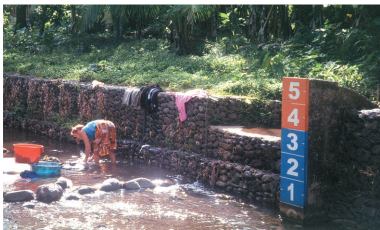
A simple flood warning system in Jamaica shows people when the water rises to danger level
