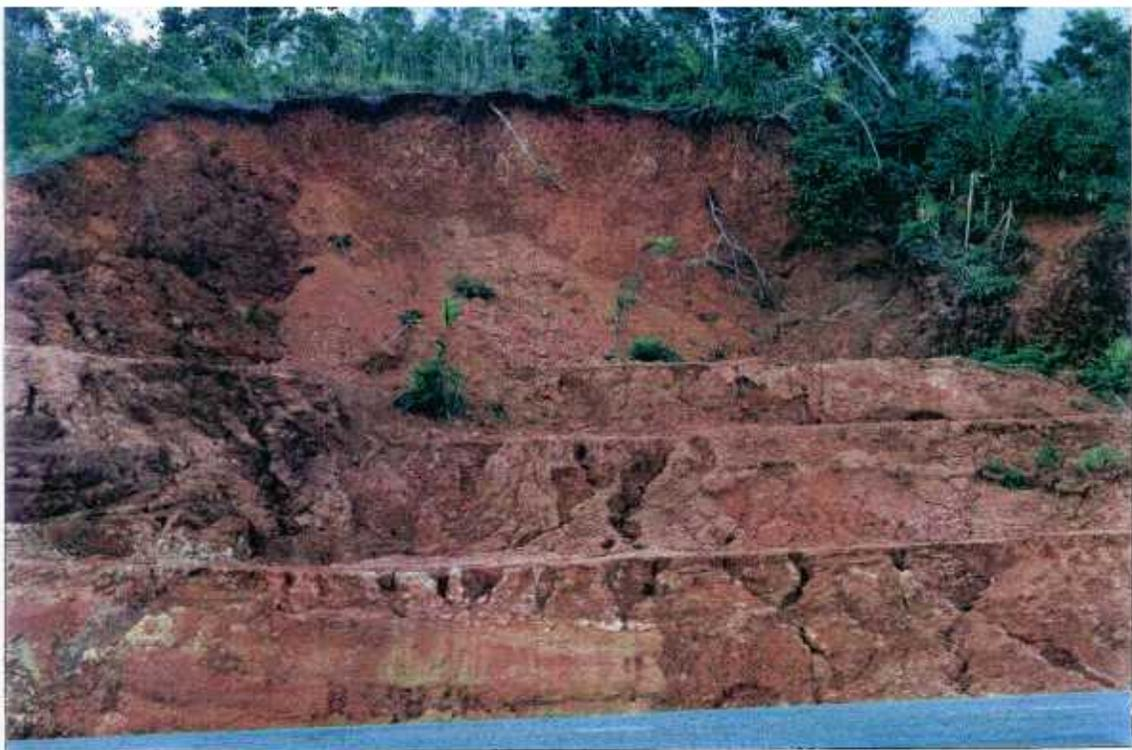
**Figure 2.10** Unstable road cutting near Galoa on the Suva-Nadi Highway. Failure is translational, involving residual soil sliding along an irregular, steeply-dipping interface with underlying weathered bedrock, and compounded by shallow rotational movements in the displaced debris mass.
