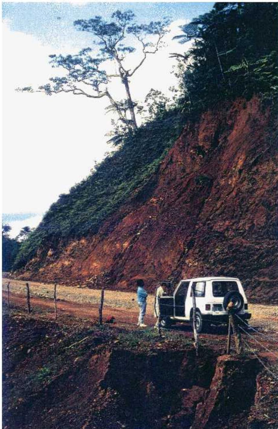
**Figure 2.8** Shallow planar translational debris slide in regolith overlying more competent weathered bedrock. Slide debris spilled onto road which has been subsequently cleared. Erosion and minor slipping in soil road fill is visible in foreground. (Location: Waindina River catchment, north east of Waivaka village)
