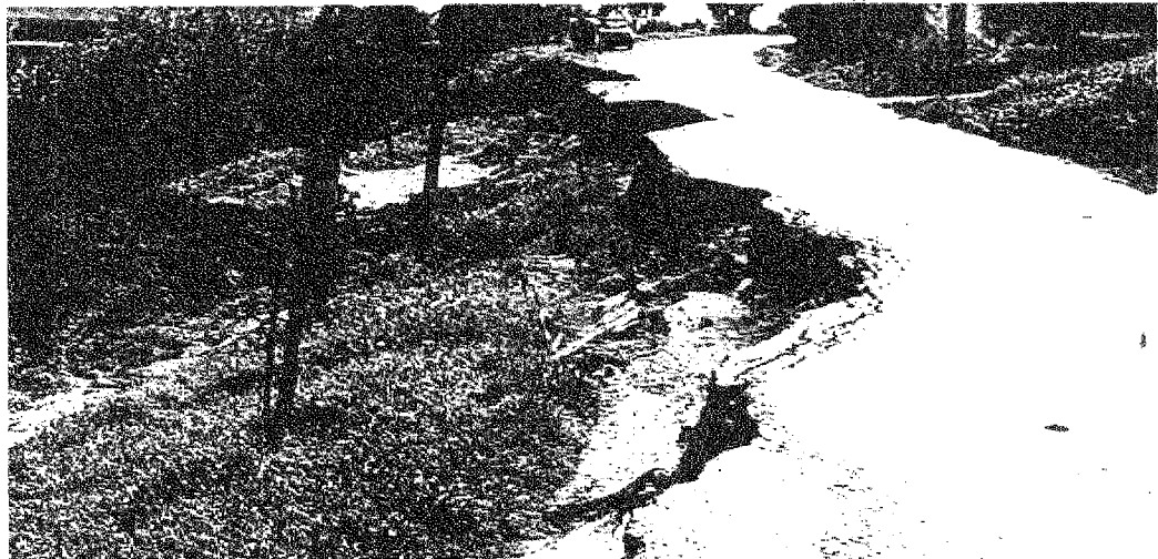
Photo 3-Road destruction by sliding at Unhos (North of Lisbon), December 1989.
