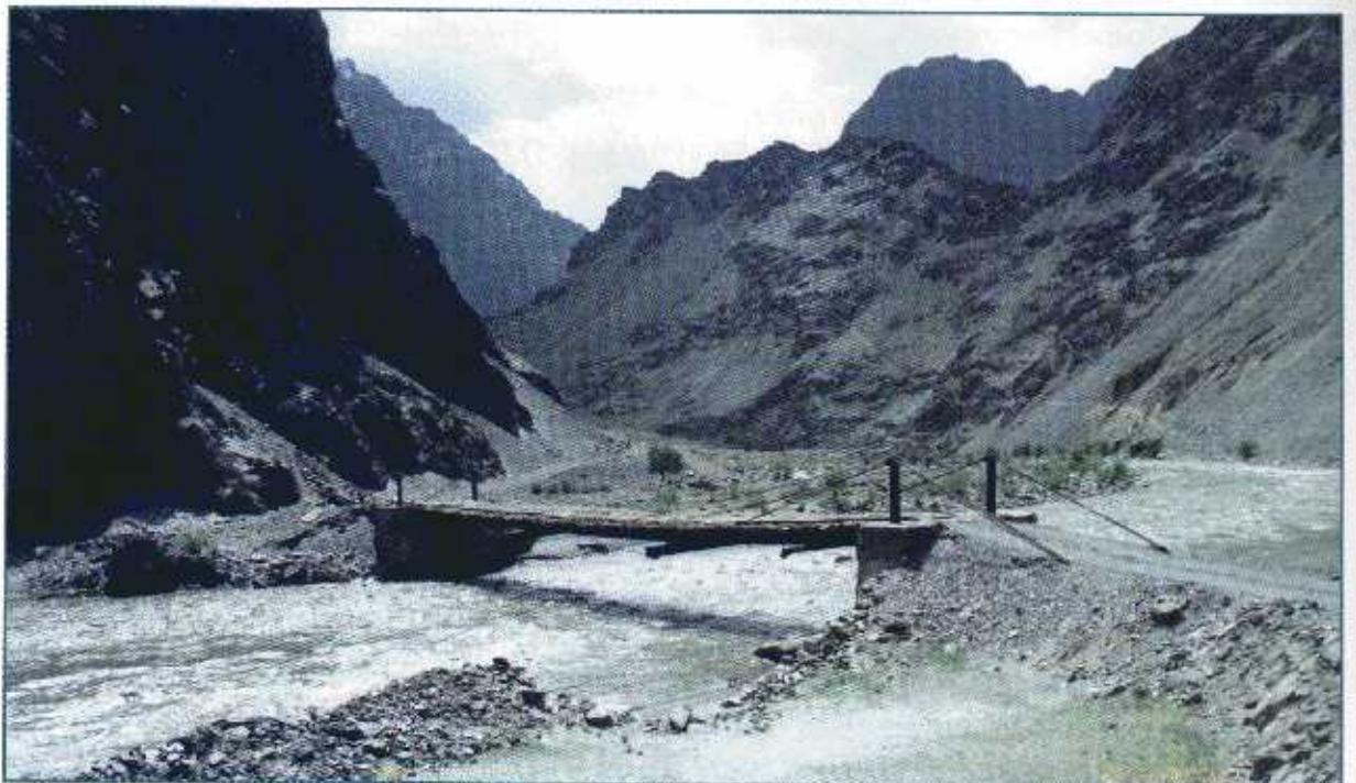
Bridge in the Bartang valley. Photo credit: Bruno Periotto.
