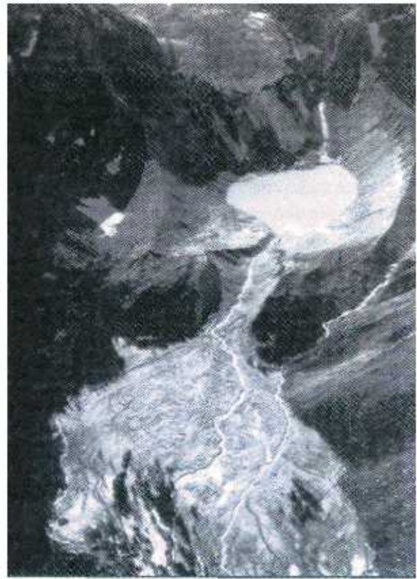
Photo 16. Typical outburst of a moraine-dammed glacier lake: A displacement wave generated by a huge ice fall overtopped the terminal moraine, surged down the steep outer face, and began eroding a narrow breach into the dam by retrogressive erosion. The lake emptied in several hours, resulting in a devastating debris flow (From Evans and Clague, 1994).
