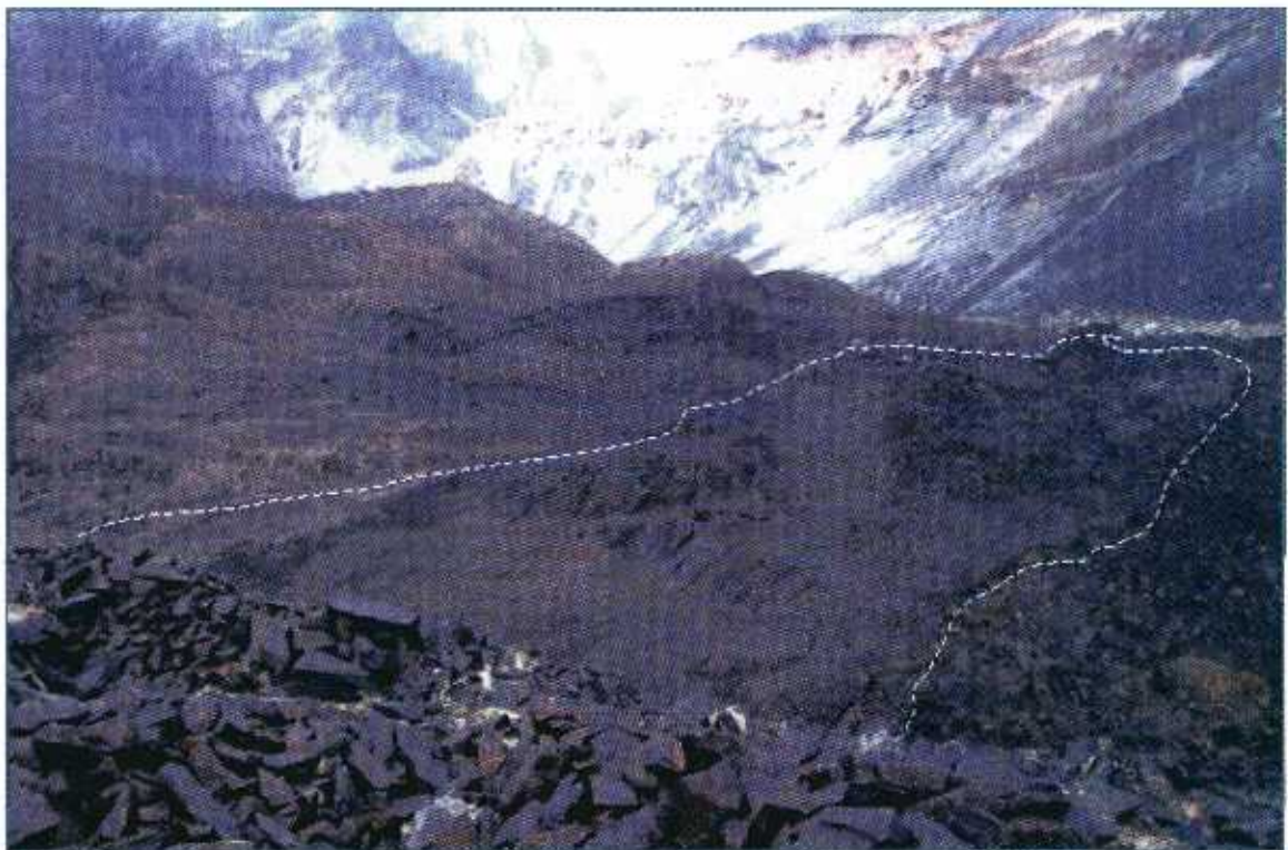
Photo 9. Huge, rather undisturbed rock block (dashed line) within the central part of the dam. This block was displaced by a secondary landslide (scarp is immediately behind the blocky material near the crest line of the dam). Photo credit: Jörg Hantsch
