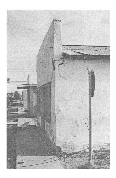
Damage to the parapet wall above the storefront opening of the warehouse (FIG.6) appears to have been concentrated in the small cross sectional area at the connection of the front and side wall. No bond beam was evident on this structure.
