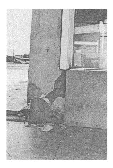
The Laundromat damage (FIG.5) was confined to the lateral movement of an unbraced wall adjacent and untied to the front wall.
