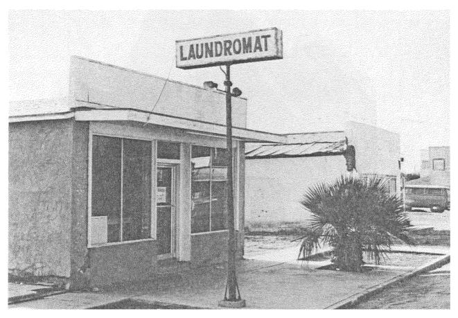
Two adobe structures, the Laundromat and an adjacent Warehouse, were moderately damaged (FIG.4). Damage was confined to the front of both of these structures, to wall sections poorly braced adjacent to storefront openings of large dimension.
