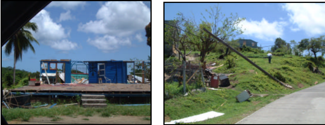
Figure 6 Damages caused by Hurricane Emily
