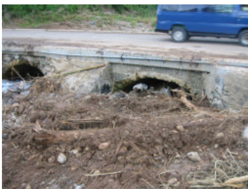
Figure 17 Debris Blockage
