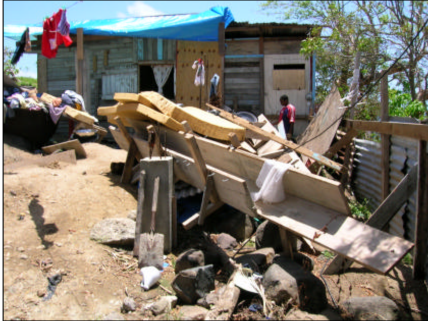
Figure 7 House Damaged by Emily. Photo Credit: OECS Secretariat
