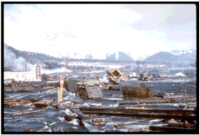
The port of Valdez, AK after the tsunami of March 27, 1964.
