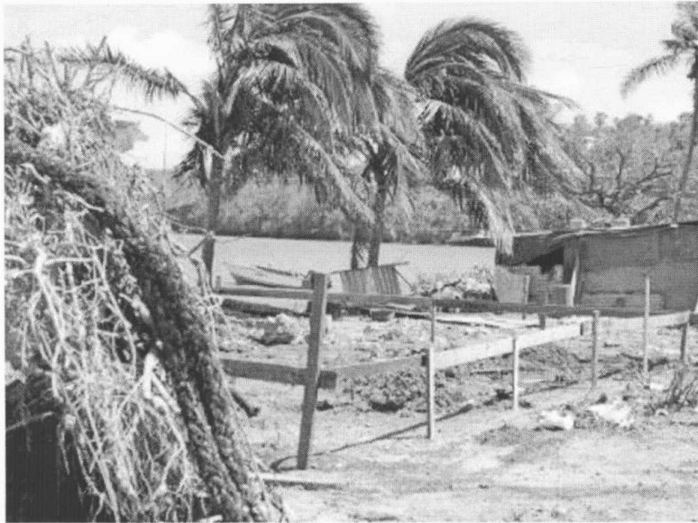
Photo 11 Reconstruction of housing at Soubise/Marquis
