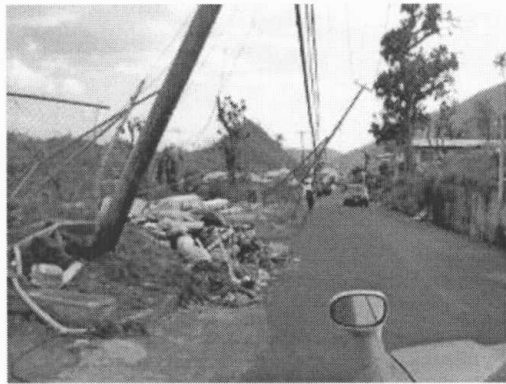
Photo 4 Typical Damage to Electric Poles
