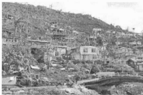
Photo 1 Damaged Housing in St. Georges
