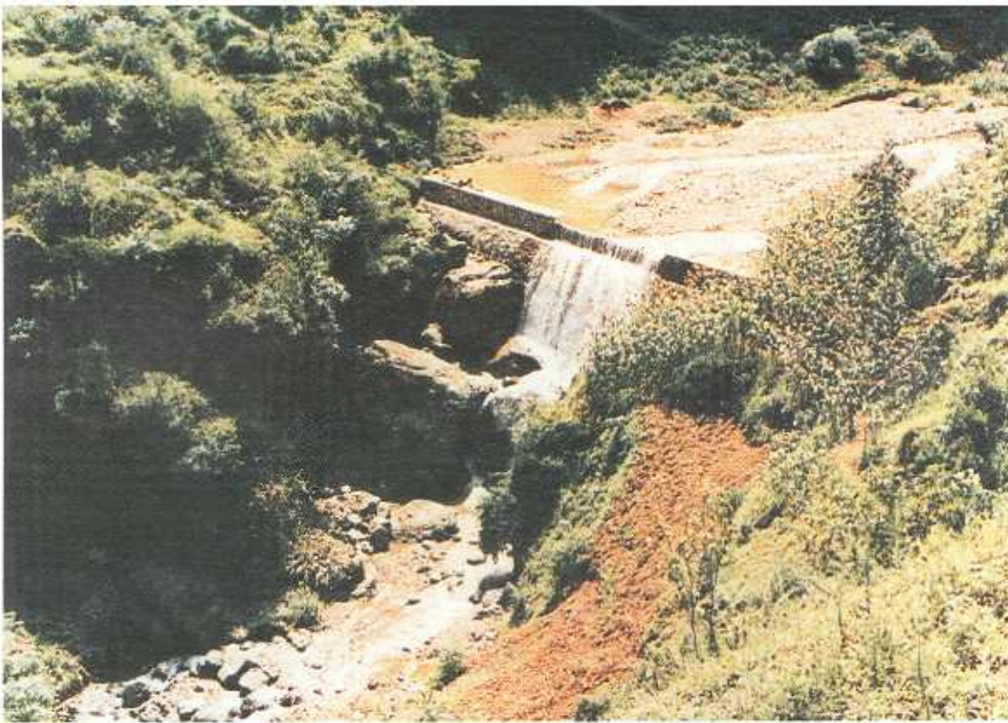
Photo 10: Structural gully control works are an effective means for the control of sediment movement
