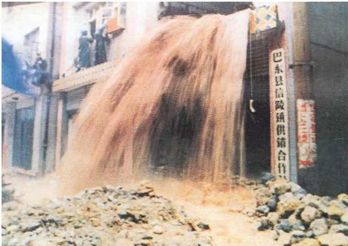
Photo 8: Mud and rock flows occur when unstable foundation material is associated with poor drainage conditions
