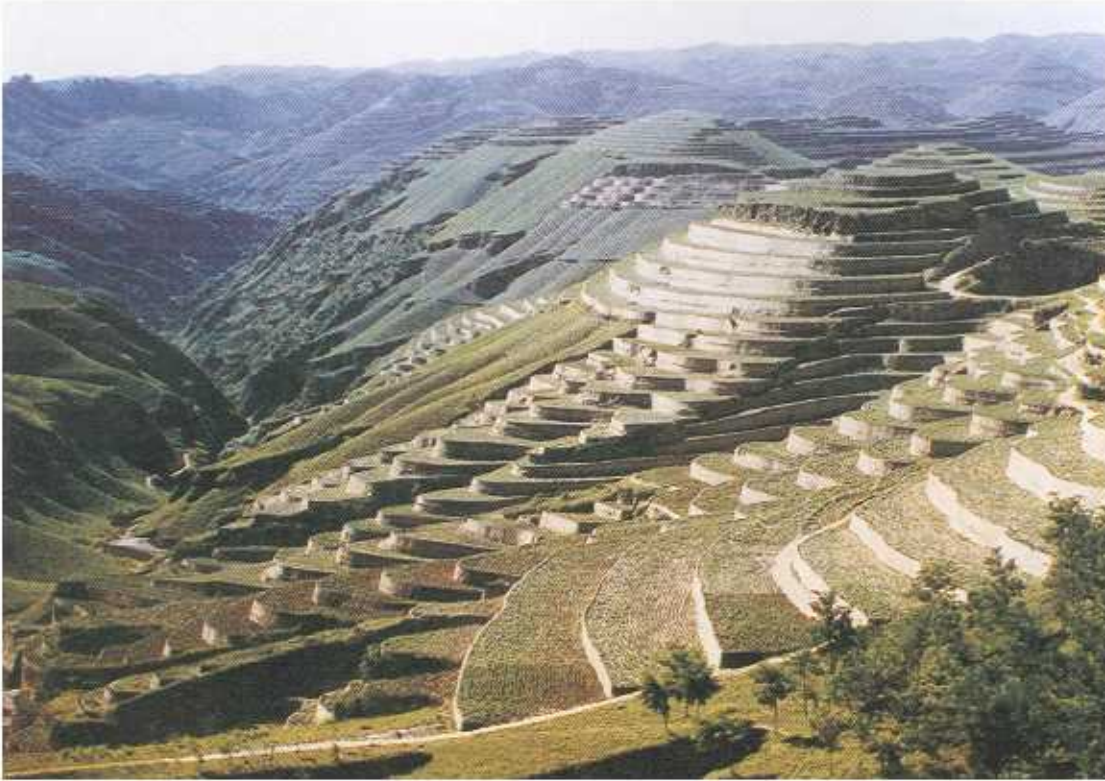
Photo 9: Dry terracing is an effective gully control measure. It is used here in the loess hills of China
