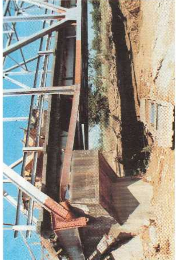
Fig. 4.21 – Damaged sections of the Dalton Pass Road at km 203 + 250 (top left) and at km 200 + 750 (top right), Courtesy of DPWH and Katahira. The collapsed Platidel Truss Bridge, over the Agno River, in Carmen (Rosales), about 60 km North of Tarlac (bottom).
