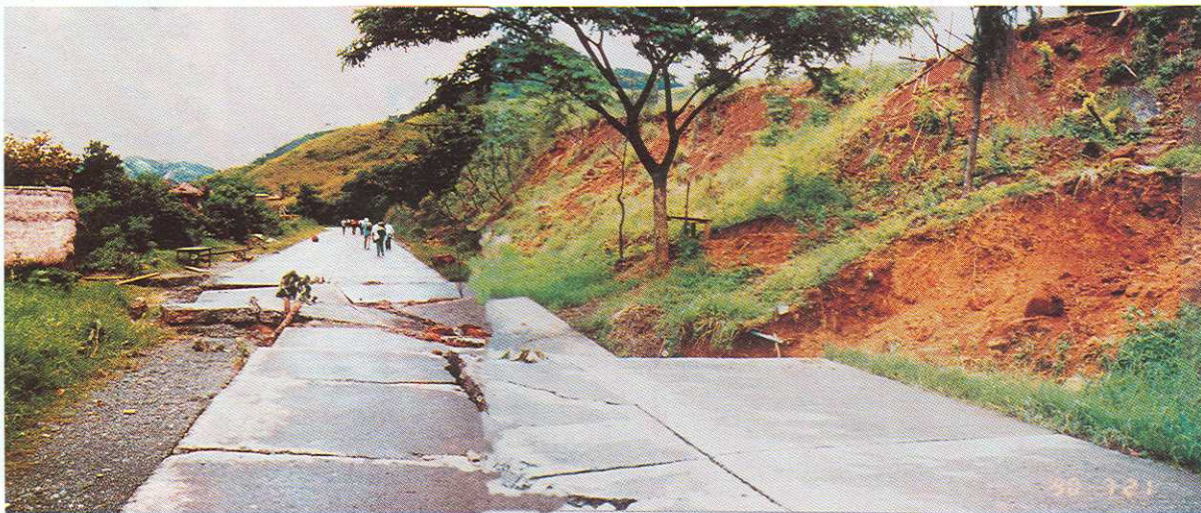
Fig. 4.15 – Fault crossing the Dalton Pass road at km 199+300 (top), at km 201+300 (center) and at km 201+400 (bottom). Courtesy of DPWH and Katahira.
