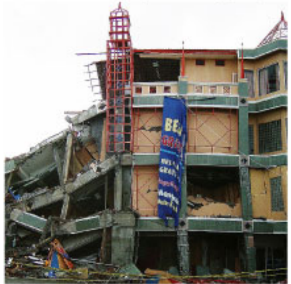
Earth Quake Damage, Leveling Shops
