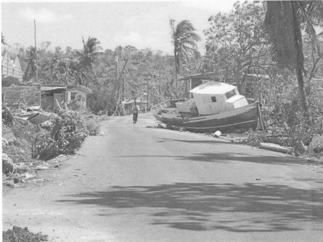
Photo 3 Damage to Soubise Area (Note boat washed onto landward side of road)
