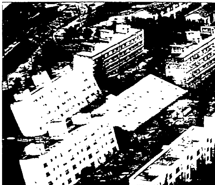
1964 earthquake, Niigata, Japan
