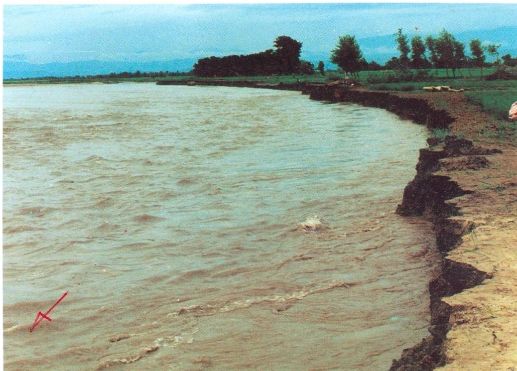
Bank cutting Kamala River
