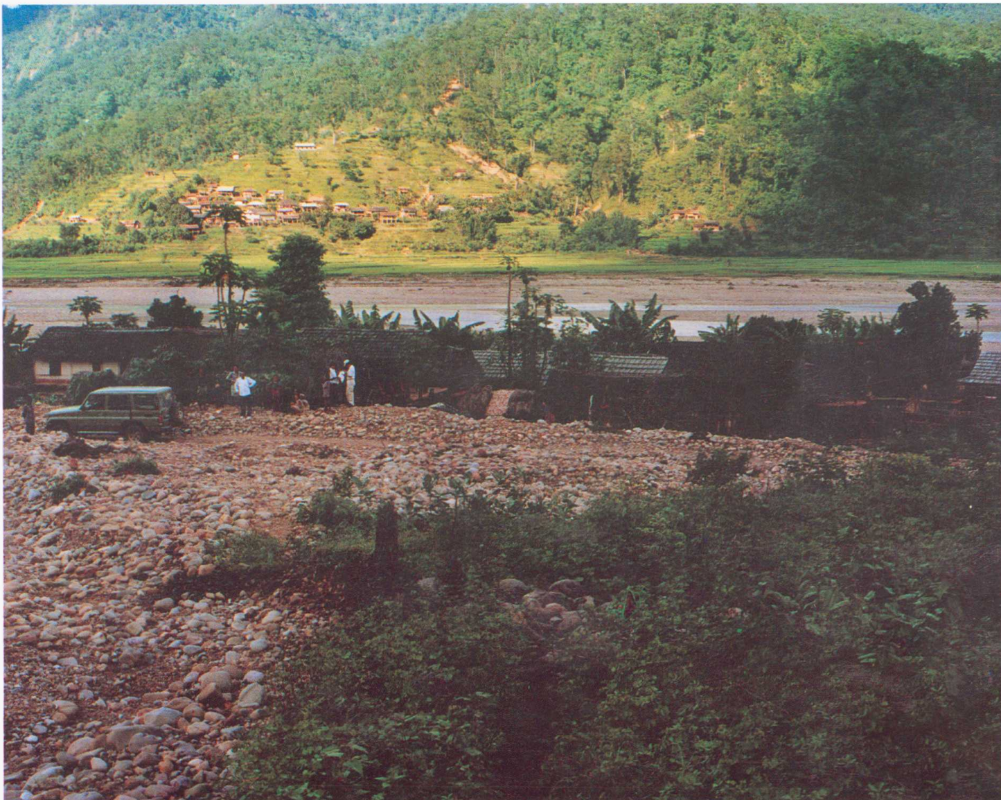
Several houses and agricultural lands were destroyed by a debris flow at Bagmara Village.
