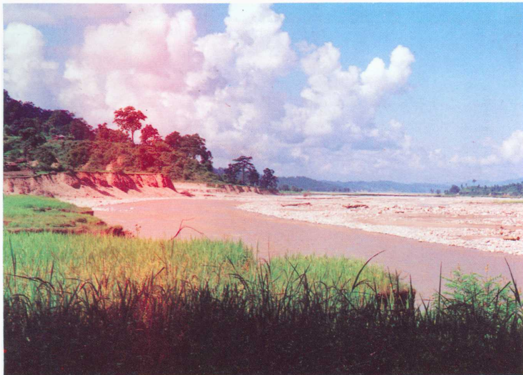
Scouring of river terrace by flood of Marin Khola.
