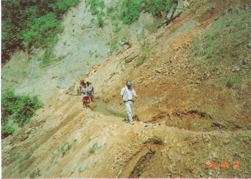
Landslide along MBT. Irrigation channel damaged by landslide in Sindhuli.
