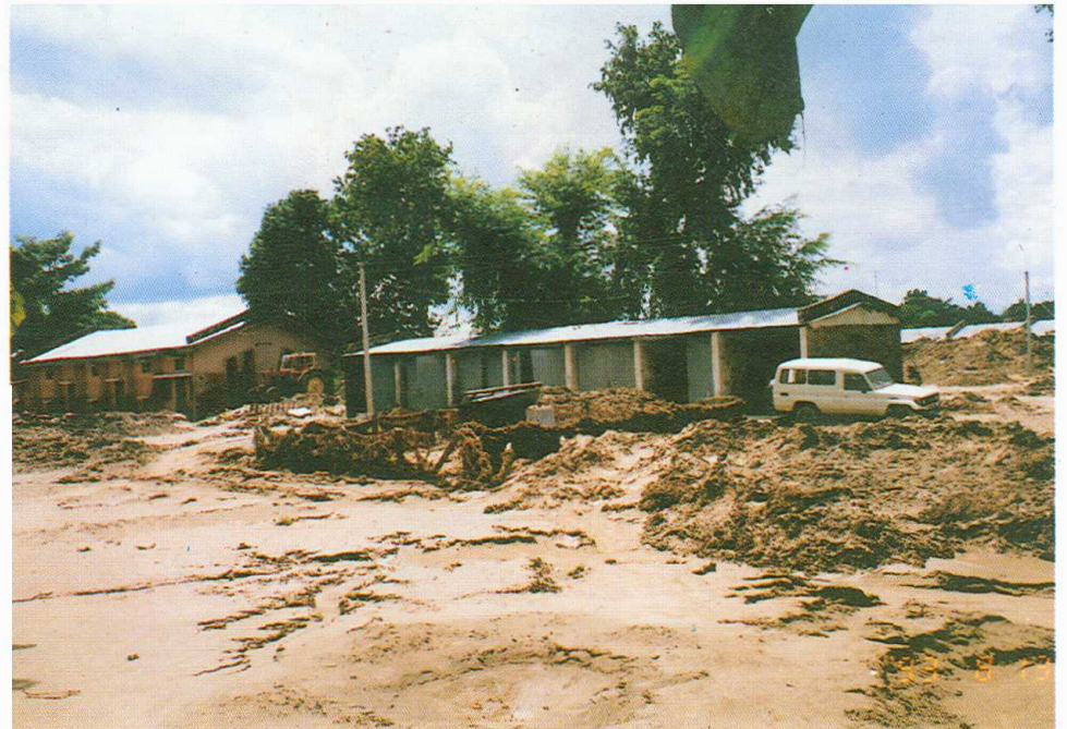
Inundation and siltation at the camp of Bagmati Irrigation Project
