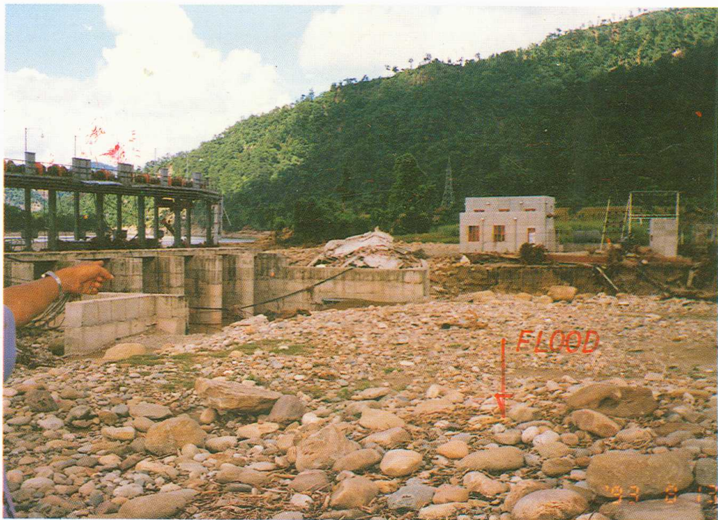
East Main Canal immediately downstream of head works.
