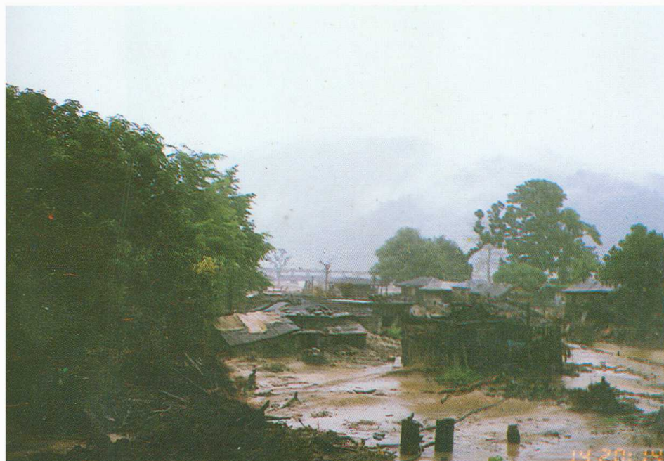
Damage to houses on the right bank of Bagmati River
