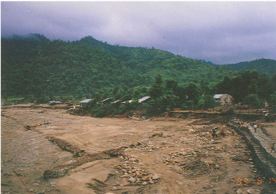
Damaged left bank between Barrage and East-West Highway
