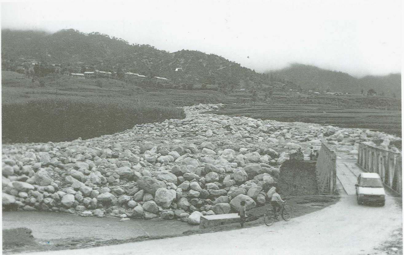
Palung Bridge narrowly escaped the attack of debris flow of Kitini Khola.
