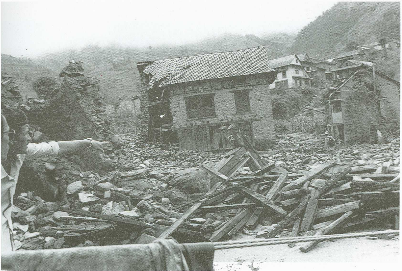
Houses wrecked in Palung by recent flood in Makwanpur.
