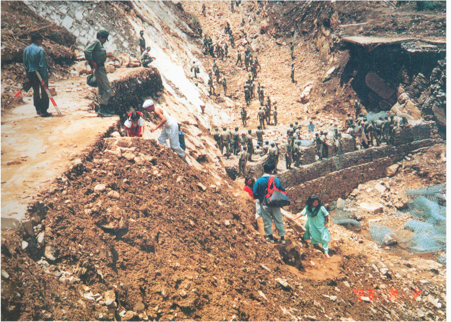
Damage to road by huge amount of debris flow at Khanigaon along Tribhuvan Highway.
