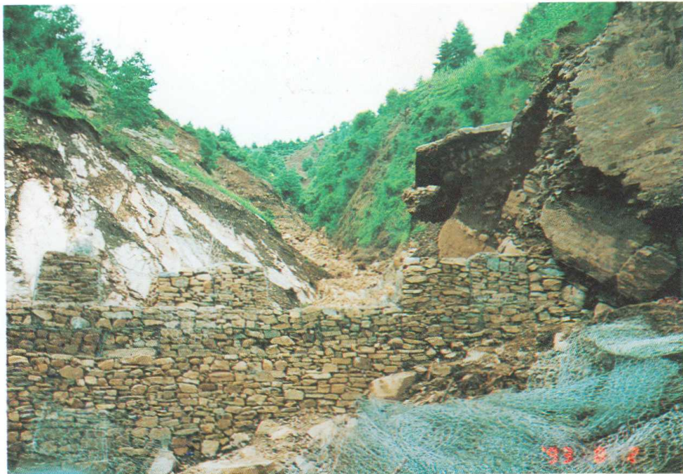
Gabion filling work by Royal Nepal Army and Department of Roads.
