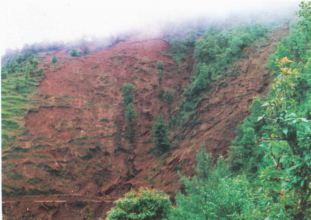
Slope failure on uphillside of Tribhuvan Highway near Malagiri, Makwanpur District.
