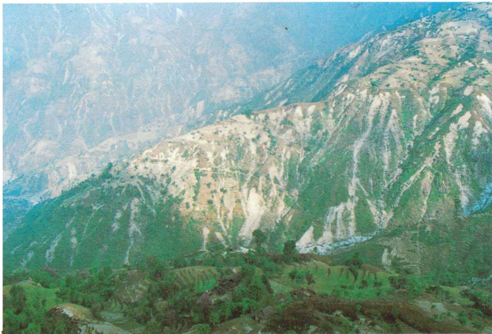
These photos show devastated situation of upstream of Agra, Belkhu and Malekhu Khola.
