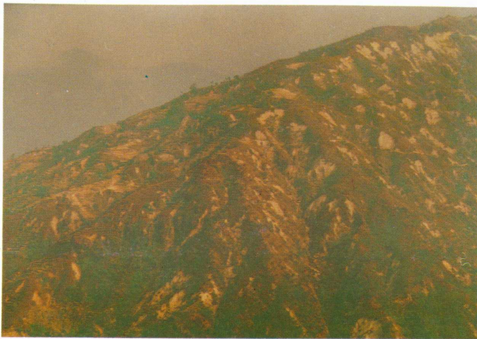
This photo shows devastated situation of upstream of Belkhu Rivers.
