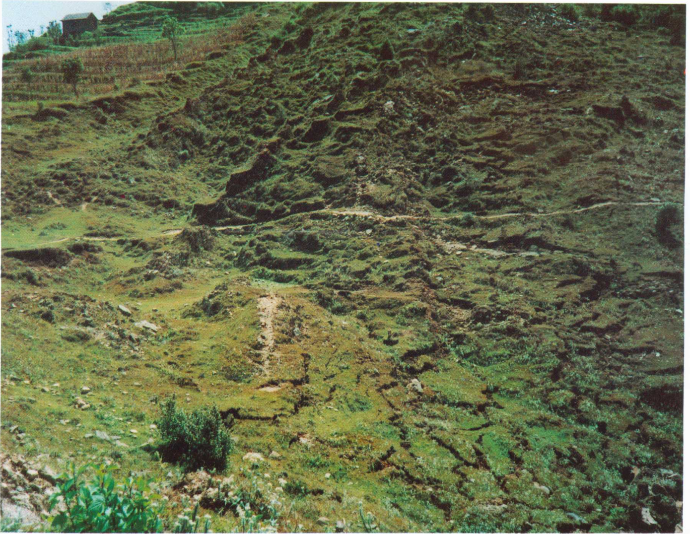
Numerous cracks at Chisapani landslide on the top of Agra Khola. Most of the cracks are observed as fresh.
