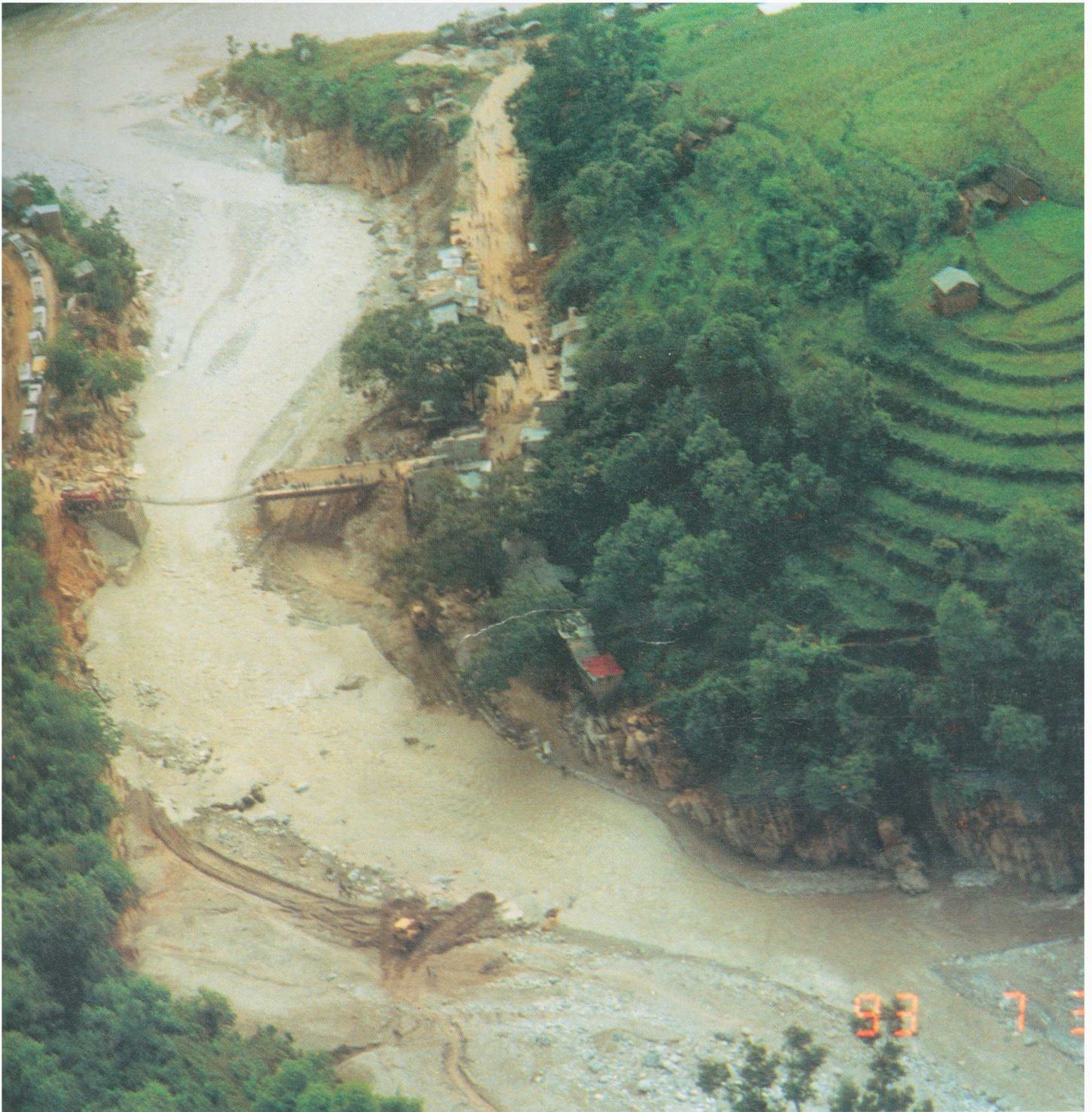
One of the decking slab of two spans Malekhu Bridge of Prithvi Highway was swept away by high flood of July 1993. The bridge had been raised by one meter when it was destroyed by floods in 1985
