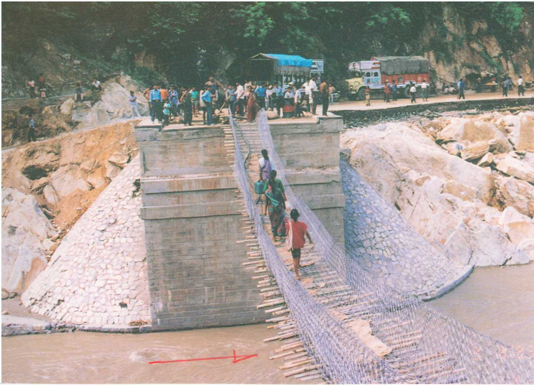
Temporary suspended crossing over Malekhu Khola
