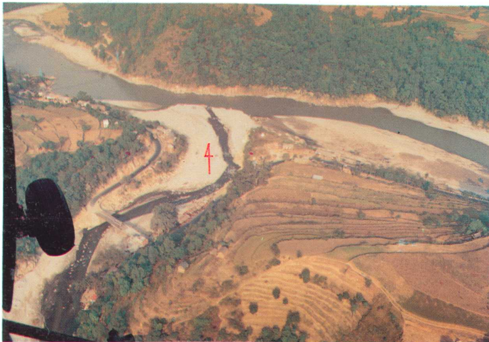
Newly established Bailey Bridge.
