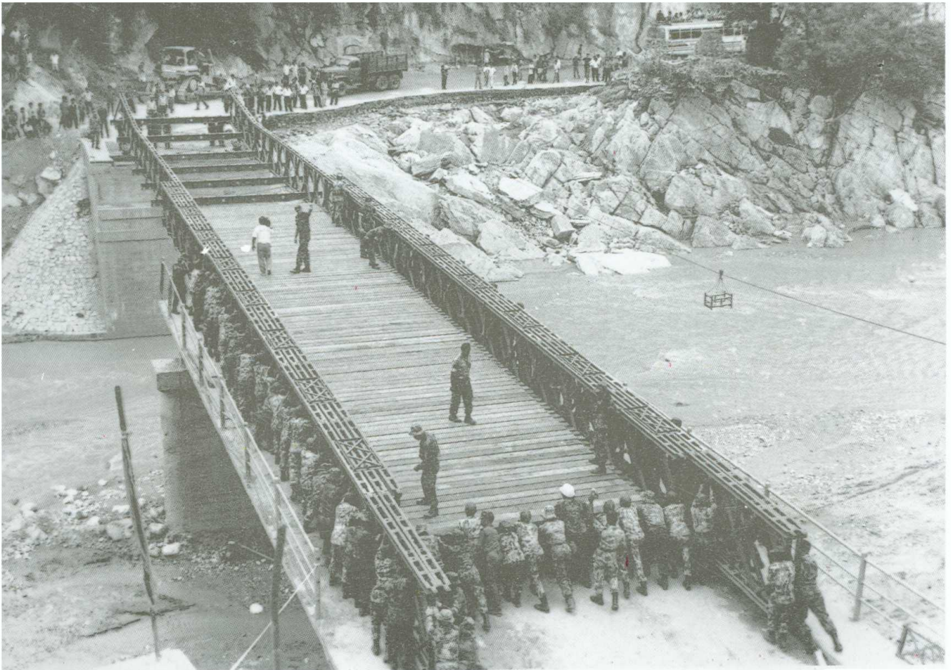
Erection of Bailey Bridge over Malekhu Khola by British Army and Royal Nepal Army.
