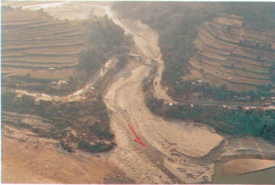
Newly established Bailey Bridge over Malekhu Khola
