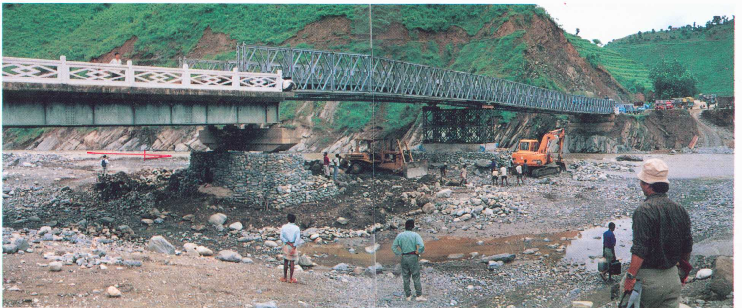
Newly established Bailey Bridge over Agra Khola at Mahadevbesi.
