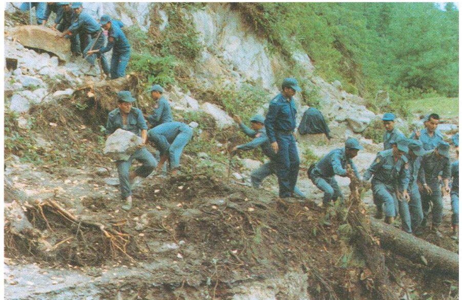
Nepal Police helping to fill boulders in gabions in Saptakoshi River on August 4, 1993.
