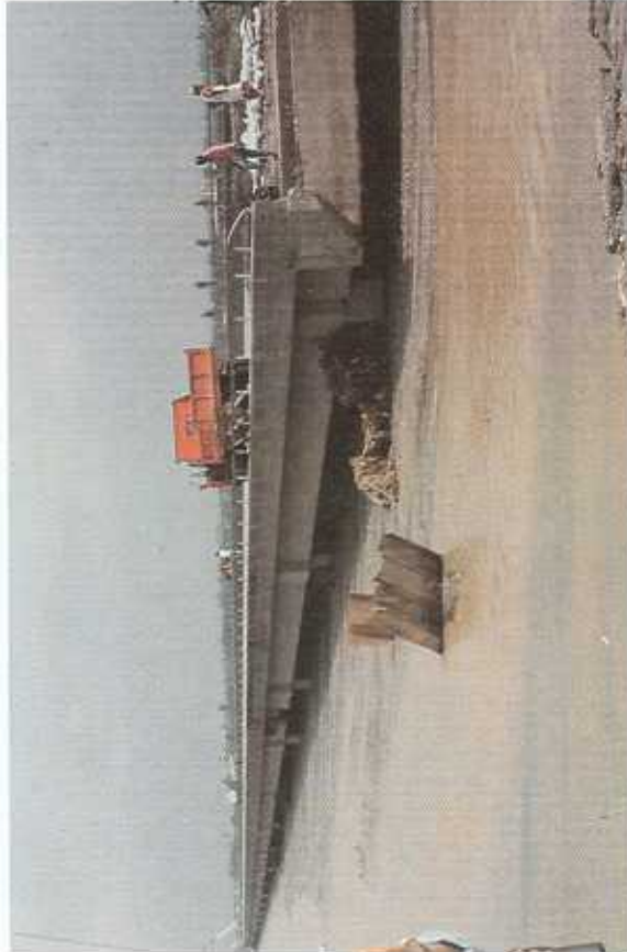
Fig. 8.14 Clogged riverbed in Tarlac (top left), and partially filled riverbed of the Bacun River (top right), on the Zambales side. Collapsed bridge span and clogged riverbed along the Superhighway around 30 km N of Manila (bottom left), and clogged floor of the Apaya River with only 1 m clearance (bottom right), north of Manila.
