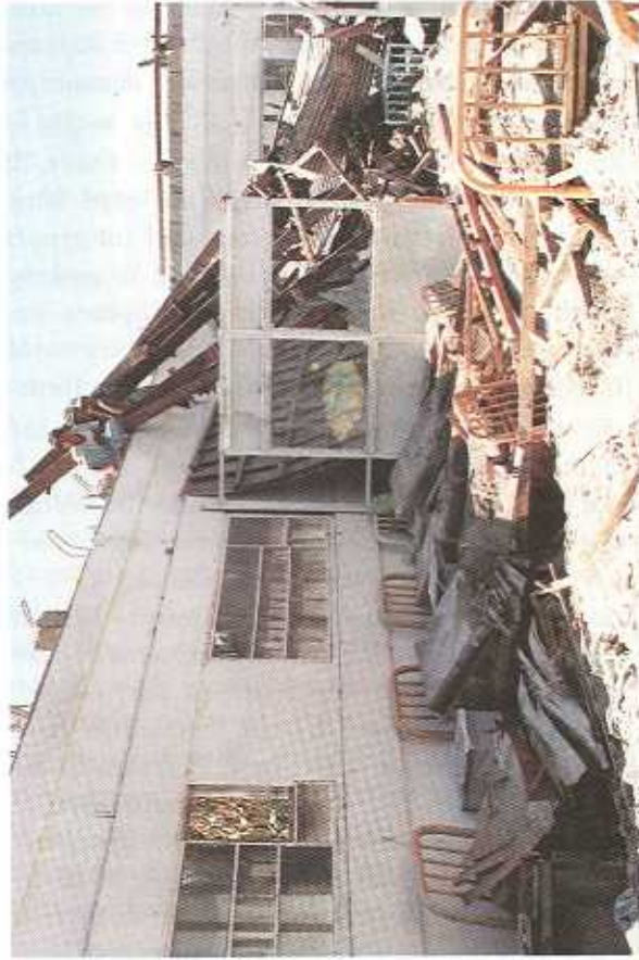
Fig. 8.11 - Collapsed school in Panau (top left), damaged roofs (top right) and destroyed hospital (bottom left) in Olongapo City, and collapsed roof in San Narciso, Zambales, (bottom right). Light roofs in general could not withstand the weight of the ash cover.
