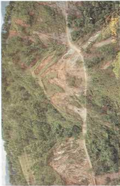
Fig. 6.7 – Shallow-seated landslides (mainly debris slides) along the road leading to Ambuklao damsite.
