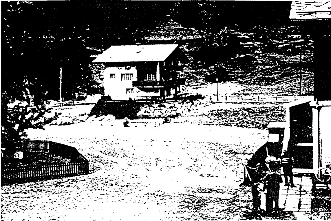
Fig.9.5 Building at Saas Balen, Switzerland, in the flood reach of Saaser Vispa. The earth fill renders it practically floodproof.
