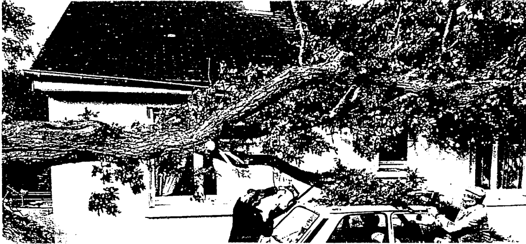
Fig.1.2 Roof damaged by falling tree during a storm.
