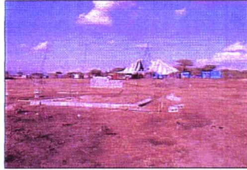
Construction has commenced at Nueva Eden
