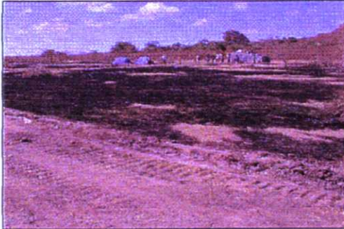
Site work has begun at Nueva Choluteca
