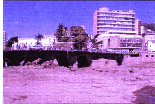
Extensive sediment deposition has greatly reduced the bridge capacities in Tegucigalpa
