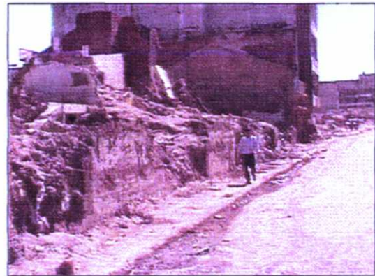
Heavy sediment deposition characterized the flooding in Tegucigalpa.
