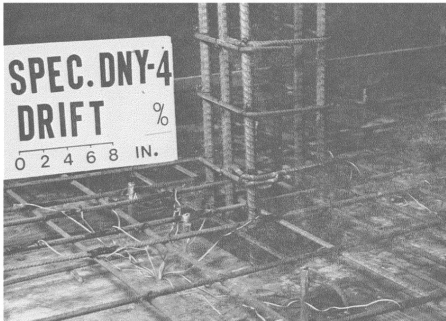
FIGURE 2-4 Interior Connection Reinforcement in DNY_4
