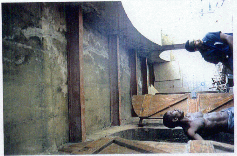
Photo 21: Inadequate hold-down detail on Baron Wing verandah.
