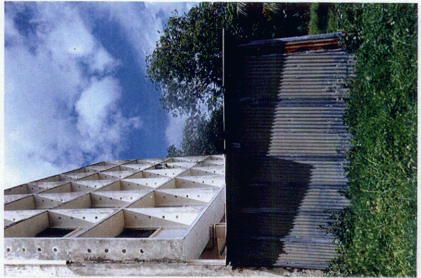
Photo 17: New infill walls constructed on the lower floor of the former nurses home.
