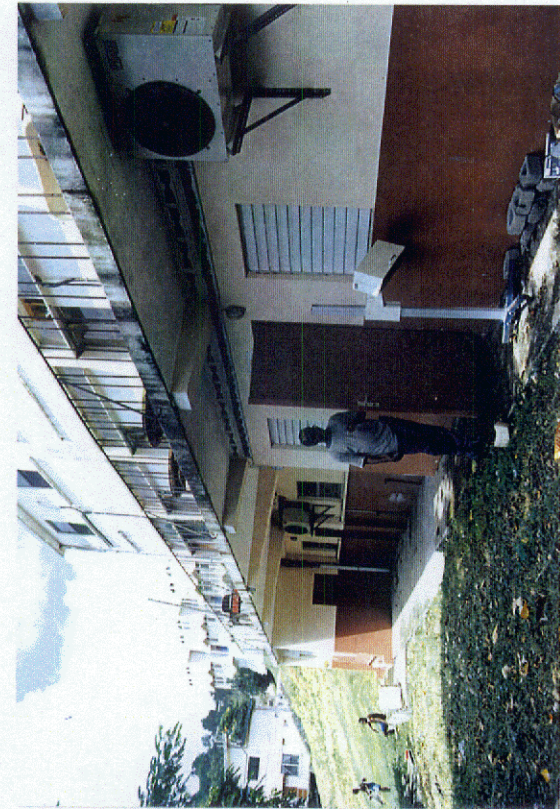
Photo 17: New infill walls constructed on the lower floor of the former nurses home.
