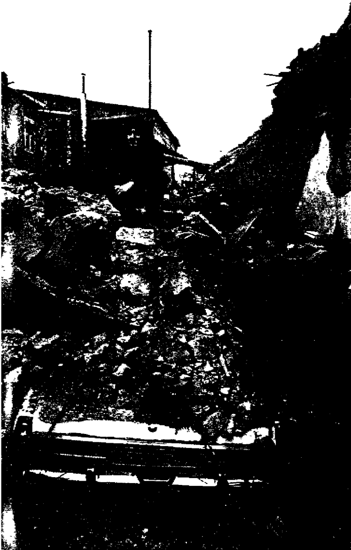
Rapidly built new constructions were first to collapse in the 1988 Spitak earthquake in Armenia
