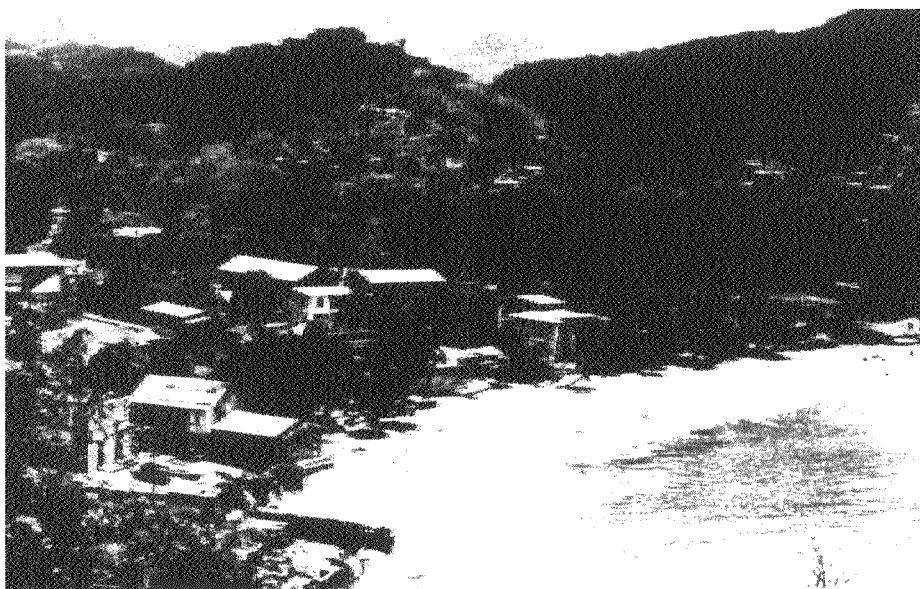
Public and private buildings close to sea-front.
